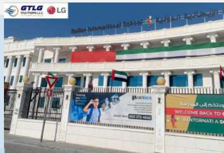
Project: ITALIAN SCHOOL, KHALIFA CITY Location: Abu Dhabi Description: Comprehensive LG air-conditioning solutions
