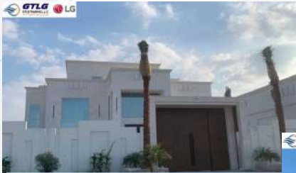
Project: PRIVATE VILLA in Abu Dhabi Description: Supply of LG Air conditioning
