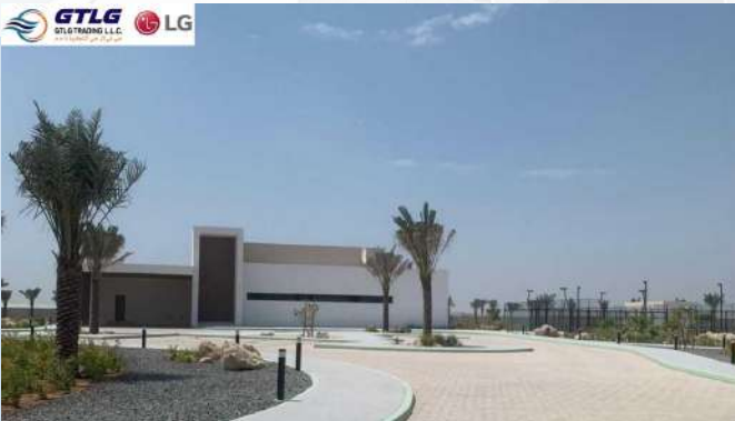
Project: PRIVATE FARM Location: Abu Dhabi Description: Supply of LG Air conditioning
