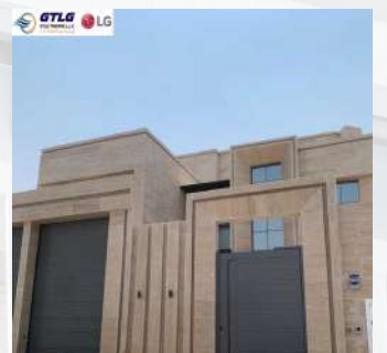
Project: PRIVATE VILLA in Abu Dhabi Description: Supply & Installation of LG Air conditioning
