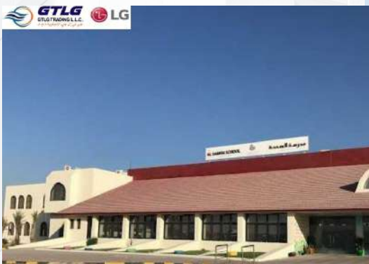
Project: AL SAMHA SCHOOL, KHALIFA CITY Abu Dhabi Description: Supply & Installation of LG air-conditioning
