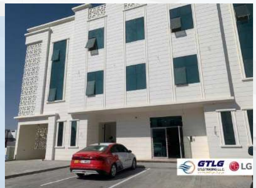
Project: "ADCE" COMMERCIAL & RESIDENTIAL BLDG Location: Abu Dhabi Description: Supply of LG Air conditioning
