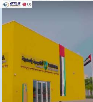
Project: ALDAR YASMINA SCHOOL, KHALIFA CITY Abu Dhabi Description: Comprehensive LG air-conditioning solutions
