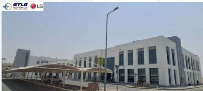
Project: ADNOC TECHNICAL ACADEMY Location: Abu Dhabi Description: Supply of LG Air conditioning
