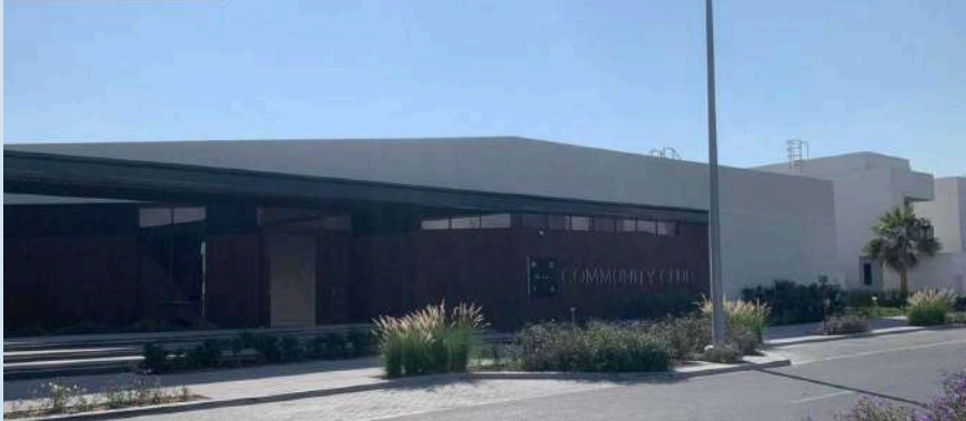
Project: NORTH YAS LIVING - COMMUNITY CENTRE Location: Abu Dhabi Description: Supply of LG Air conditioning
