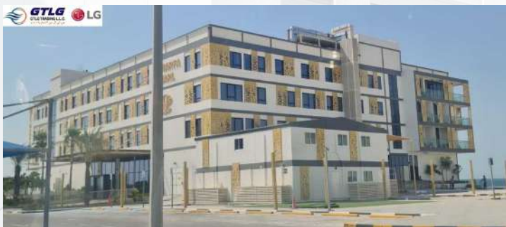
Project: AL MIRFA PEARL HOTEL Location: Abu Dhabi Description: Supply of LG Air conditioning
