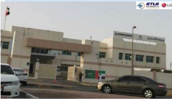
Project: AL HOSH SCHOOL, SHAMKHA Abu Dhabi Description: Supply & Installation of LG air-conditioning
