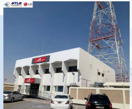
Project: ETISALAT MADINAT ZAYED Location: Abu Dhabi Description: Supply of LG Air conditioning
