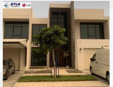
Project: PRIVATE VILLA in Abu Dhabi Description: Supply of LG Air conditioning
