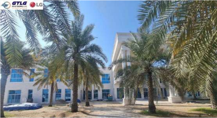
Project: AL BUSTAN PALACE Location: Abu Dhabi Description: Supply of LG Air conditioning
