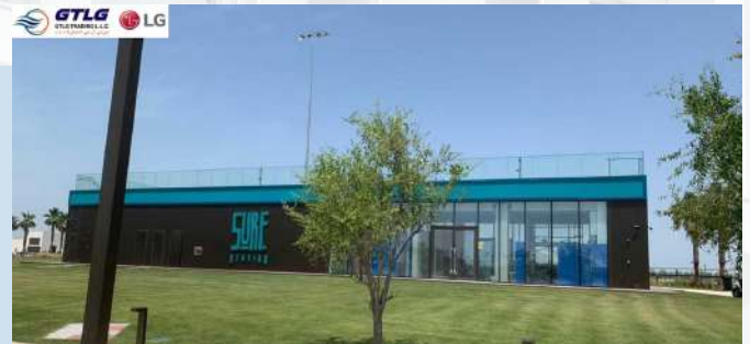
Project: SURF RANCHES, AL BATEEN Location: Abu Dhabi Description: Supply of LG Air conditioning
