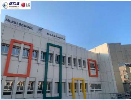
Project: MLEIH SCHOOL Location: Abu Dhabi Description: Supply of LG Air conditioning
