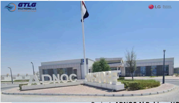
Project: ADNOC Al Dabiyya HQ Location: Al Dabiyya, Abu Dhabi Description: Supply and Installation of LG Air conditioning
