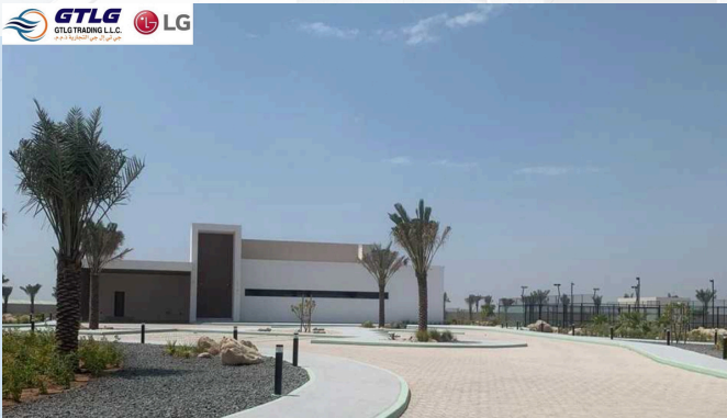
Project: PRIVATE FARM Location: Abu Dhabi Description: Supply of LG Air conditioning
