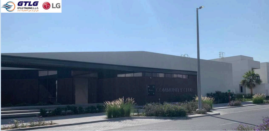
Project: NORTH YAS LIVING - COMMUNITY CENTRE Location: Abu Dhabi Description: Supply of LG Air conditioning
