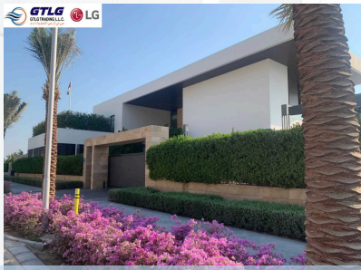
Project: PRIVATE VILLA in Abu Dhabi Description: Supply of LG Air conditioning
