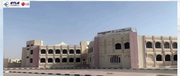
Project: AL FADHEL SCHOOL AL AIN Location: Al Ain, Abu Dhabi Description: Supply of LG Air conditioning
