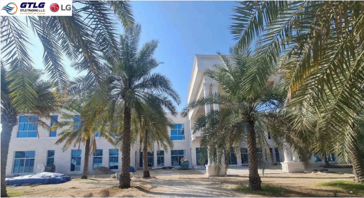
Project: AL BUSTAN PALACE Location: Abu Dhabi Description: Supply of LG Air conditioning
