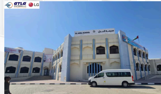
Project: AL ADEL SCHOOL AL AIN Location: Al Ain, Abu Dhabi Description: Supply of LG Air conditioning
