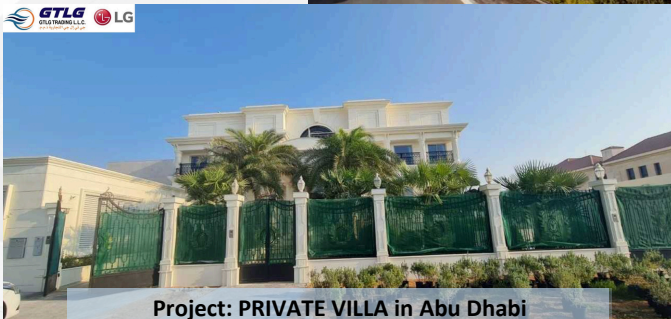
Project: PRIVATE VILLA in Abu Dhabi Description: Supply of LG Air conditioning
