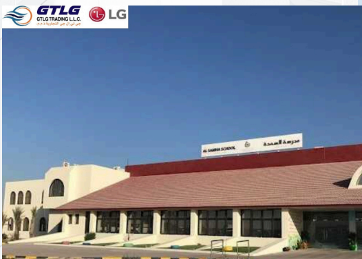
Project: AL SAMHA SCHOOL, KHALIFA CITY Abu Dhabi Description: Supply & Installation of LG air-conditioning
