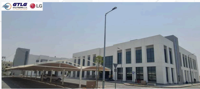
Project: ADNOC TECHNICAL ACADEMY Location: Abu Dhabi Description: Supply of LG Air conditioning
