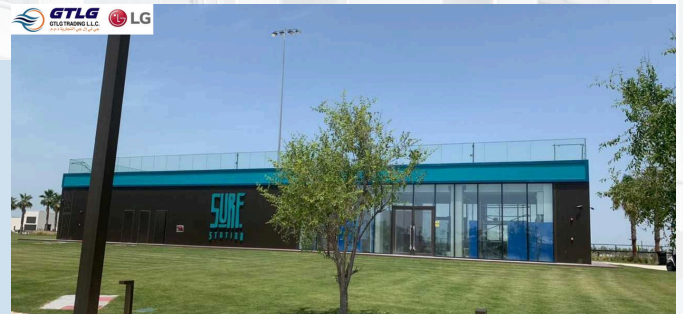
Project: SURF RANCHES, AL BATEEN Location: Abu Dhabi Description: Supply of LG Air conditioning
