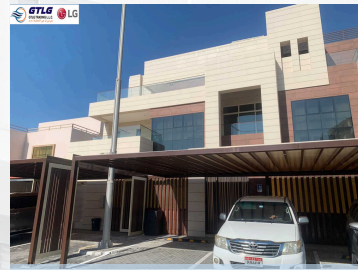
Project: PRIVATE VILLA in Abu Dhabi Description: Supply & Installation of LG Air conditioning
