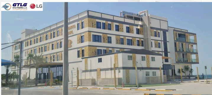
Project: AL MIRFA PEARL HOTEL Location: Abu Dhabi Description: Supply of LG Air conditioning
