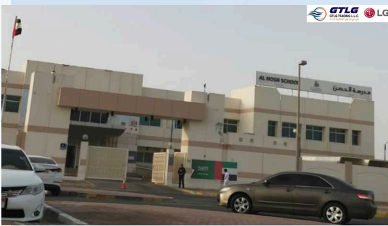
Project: AL HOSN SCHOOL, SHAMKHA Abu Dhabi Description: Supply & Installation of LG air-conditioning
